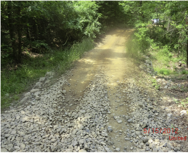
Fig. 5. Downhill concentration of rock fragments due to dry ravel.
