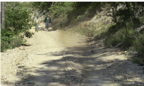
Fig. 6. Cobble and gravel sorting by wheel ravel.
